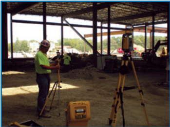
K-B Foreman Tracy Olkiewicz uses Trimble MEP Layout Solution at the Des Plaines Casino jobsite
